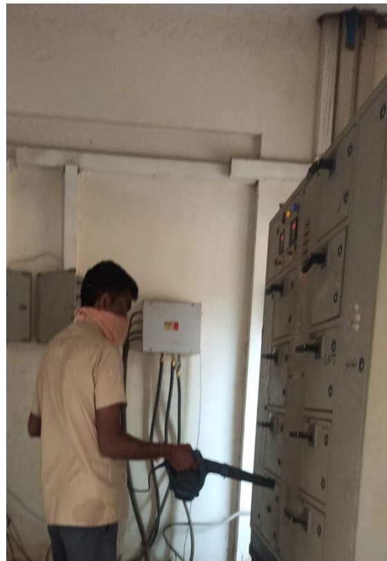
Cleaning Electrical panel boards
