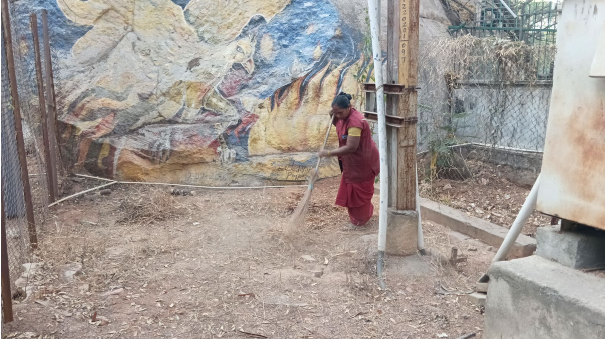
Cleaning 11KV CTPT yard
