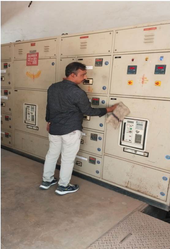
Cleaning Electrical panel boards
